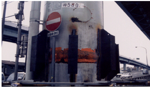
Fig. 1. Local buckling of steel bridge pier, Kobe Earthquake, January 1995.
