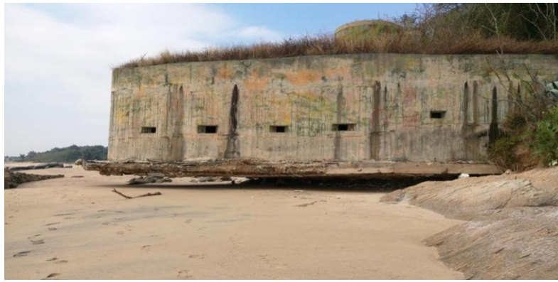
Figure 3. Photo of a Coastal Military fortress showing eroded foundation. (Kao et al, 2017)
