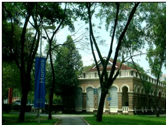
Fig. 8. Conservation of Sentul Warehouse into design
