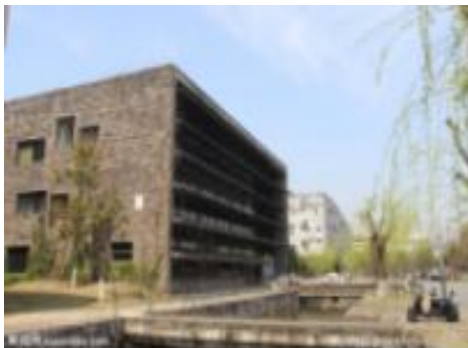
Figure 3 No.12 Xiangshan Campus, CAA
